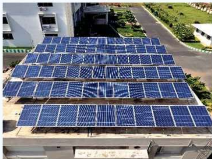
110 kW of roof-top grid connected Solar Power, Green plantation, and Rainwater harvesting
