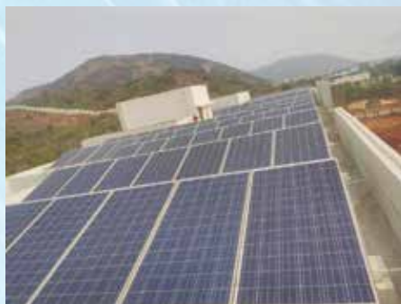
Installed 60KW Solar Power on Building terrace at SAMEER, Visakhapatnam
